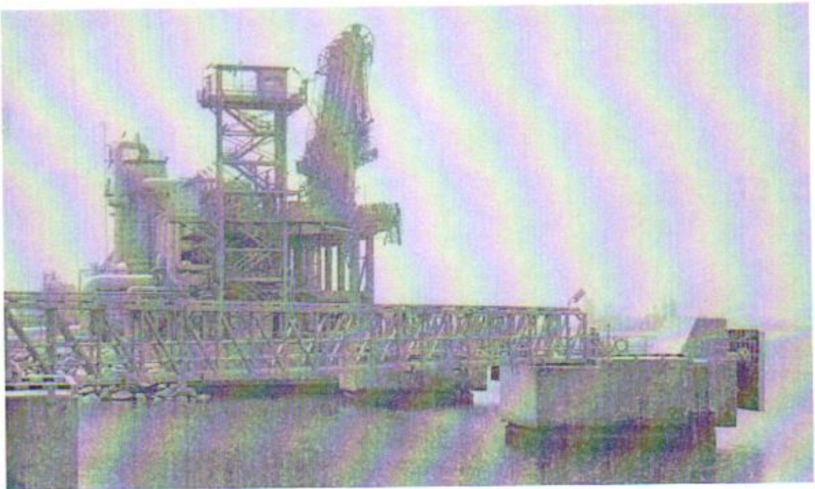
LNG Berth 2 - Loading Platform and Breasting Dolphins
