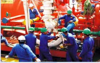
Technical staff attach the liquid and vapour lines for transfer of product from a gas carier at LPG terminal
