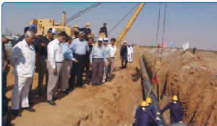
Transmission line being lowered in trench
